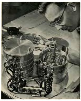
Last edition's 'Fifty+ Years Ago' image showed a CSIRO experiment designed for launching in a satellite, to measure the presence of VLF radio waves. It's reported that the equipment, built in 1962, cost £500 for material alone! Nowra was used for testing the device, using the Met Section's weather balloons to a height of 200,000 feet. Nowra was also chosen because of the lack of radio noise, particularly when the 'Pundit' was turned off and there was no night flying.
