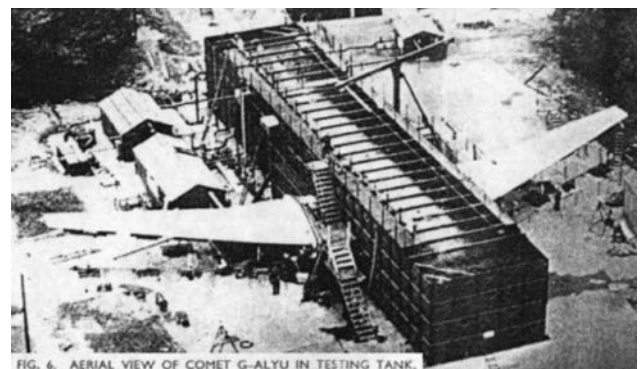
FIG. 6. AERIAL VIEW OF COMET G-ALYU IN TESTING TANK.
