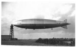
The R101 was to carry 100 passengers with an endurance of 57 hours at a cruise speed of 63 knots. In wartime, the airships were expected to carry 200 troops or possibly five deployable fighter aircraft.
