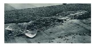
The final report of the Court of Inquiry was presented on 27 March 1931. Various theories of the cause of the crash were tested and discounted, with the Inquiry reaching the conclusion that a catastrophic tear had probably developed in the forward cover, which in turn caused one or more of the forward gasbags to fail.
