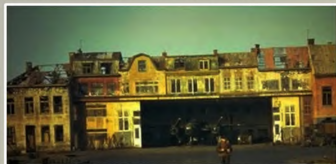
Sometimes the camouflage worked in the other way, as in this image where a real, operating aircraft hangar was shrouded in faux French chalets to hide the real purpose of the structure. The Allies used it after D-day for their own aircraft - in this case a B-25 bomber.
