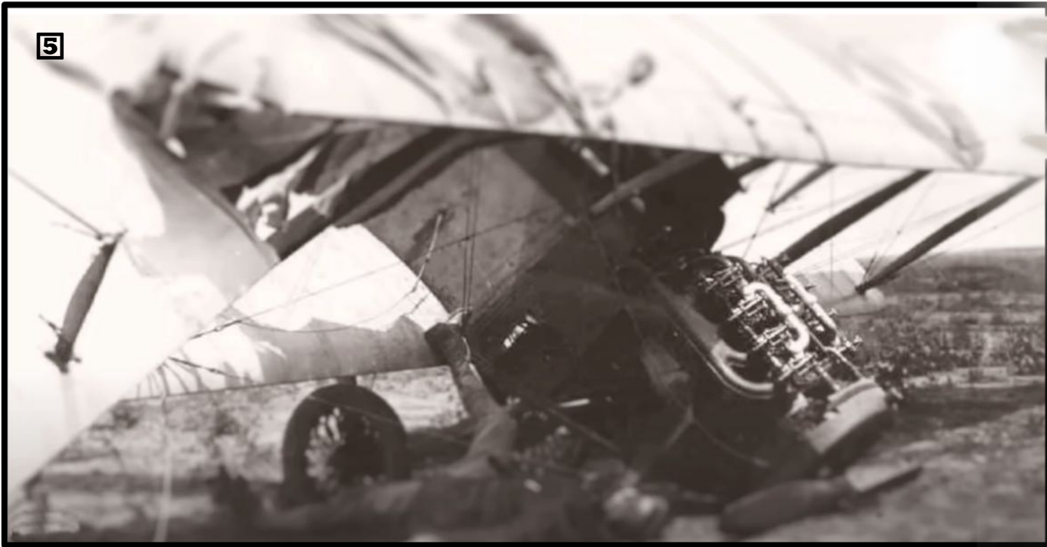
The dangers of air to air refuelling were graphically illustrated a month later, however, when this aircraft [5] crashed at an air show in Kellyfield (Texas), whilst demonstrating the manoeuvre. The hose had struck the propeller of the receiving aircraft, making it the first fatal air-to-air refuelling accident. Because of this, and the practical difficulties of dangling a trailing hose to connect aircraft together, in flight refuelling was largely regarded as a stunt.
